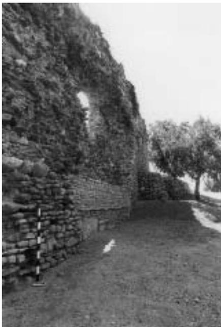
**Fig. 14: Building A (Fig. 1, no. 27), north wall, after partial infilling to replaces losses in original (Late Roman) mortared rubble and brick construction. View looking southwest**
